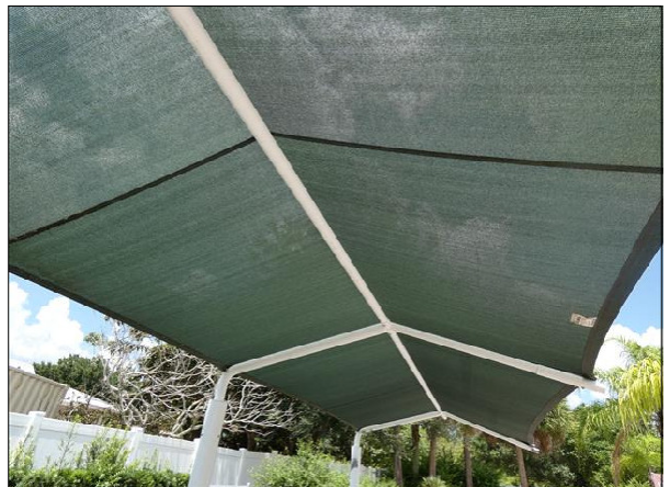
Swim Club Shade Structure
