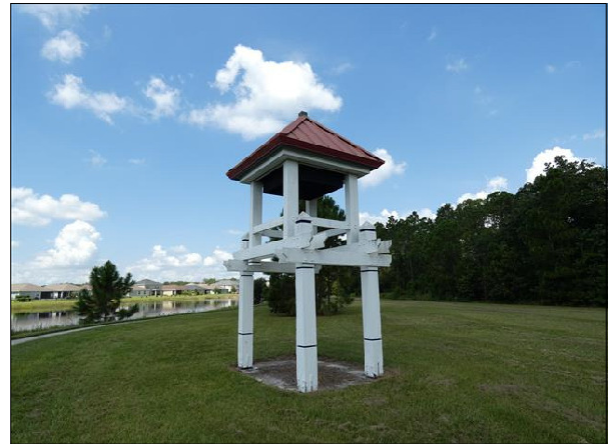
Lake Recreation Area West Pavilion
