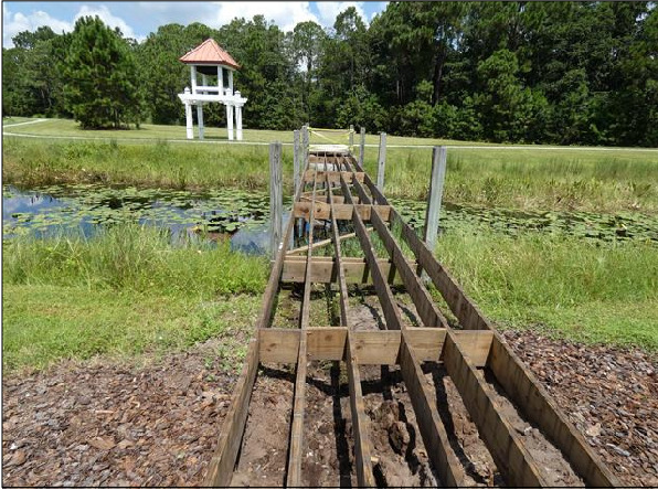
Lake Recreation Area Pedestrian Bridge
