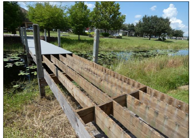
Lake Recreation Area Pedestrian Bridge
