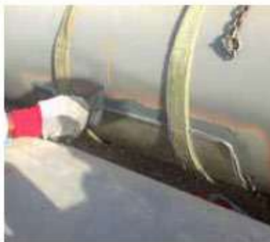
Bonding and shimming
