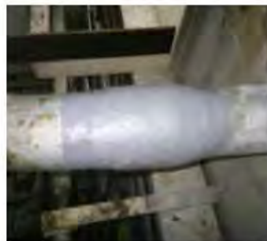
Wrapping and patching
