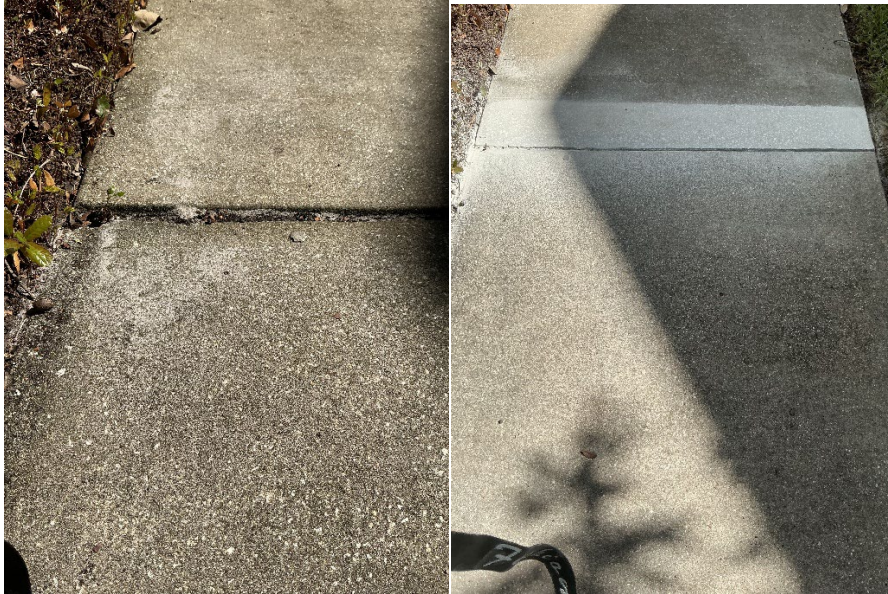
Continued sidewalk grinding on Five Oaks.
