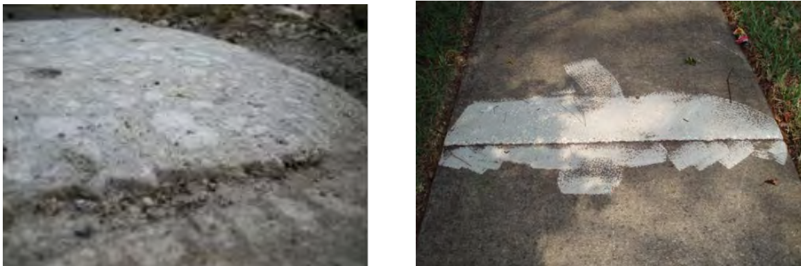
Figure 9: Typical Results from a Grinder
